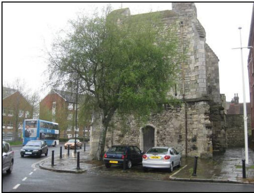
Photo 2.3: tree T4 (north side of road)
